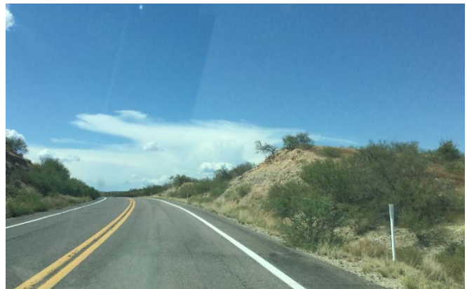
Figure 41: Slight curve delineated with object markers.
