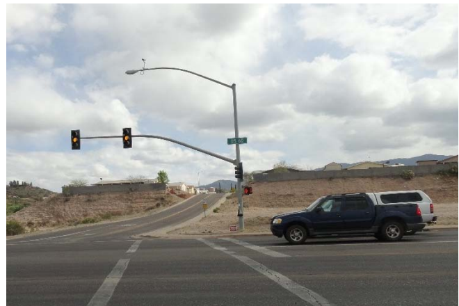
Figure 3: Faded Striping & View of Signal Heads
