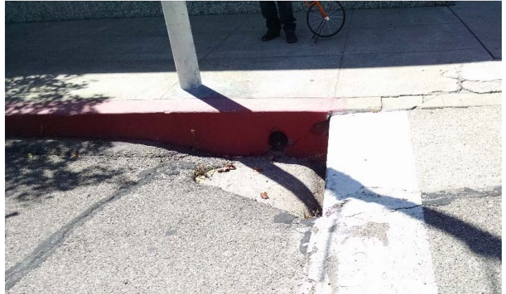
Figure 24: Inlet on southeast quadrant.
