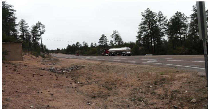
Figure 21: Ditch near Highland Drive.
