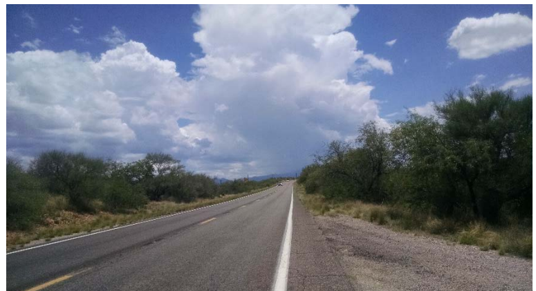
Figure 44: Vegetation close to roadway. Near a pullout.
